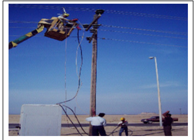
Figure 4. Connection of a conductor to one phase
